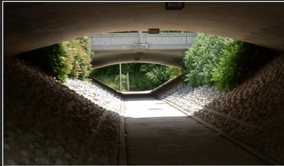
Pedestrian Bridge under Franklin Boulevard
